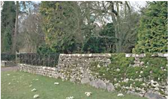
Garden wall, railings and gate to Town Head House - Grade II
