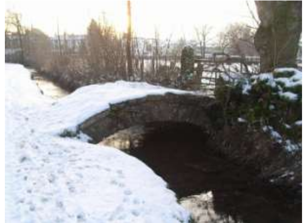
Bridge over Chapel Beck
