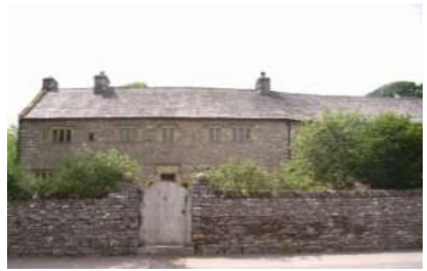
Limestone walls, often rendered and/or painted Westmorland green and Burlington blue roof slates Building lines set back from road outside of village core
