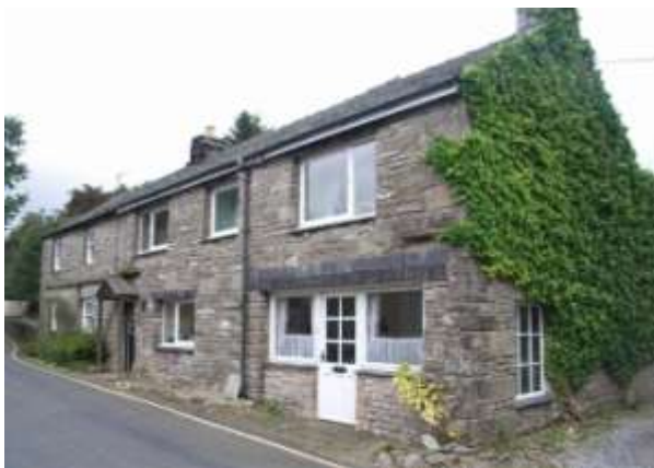
Building frontages facing road Predominance of two storied buildings
