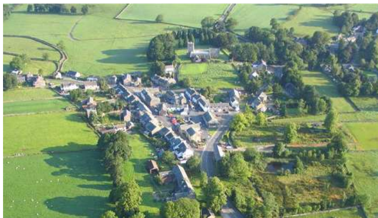
Aerial view of Orton showing All Saints church and historic village core
