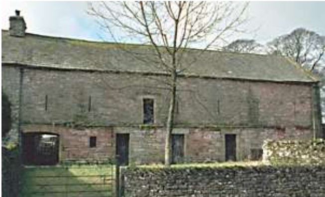
Barn and Byre Range Adjoining North End Of Petty Hall - Grade II
